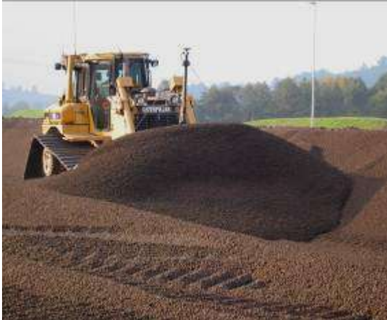
Figure 10 Spreading by dozer
