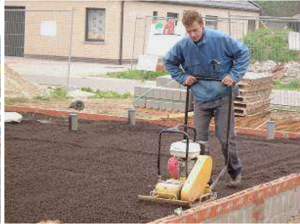
Figure 13 Compaction by vibrating plate
