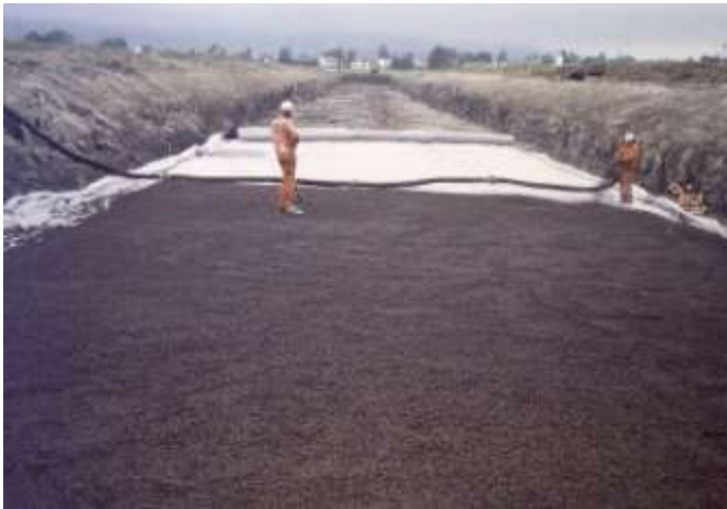
Figure 8 Installation by blowing
