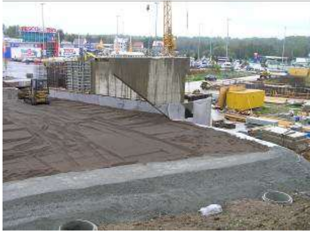
Figure 12 Compaction by dozer
