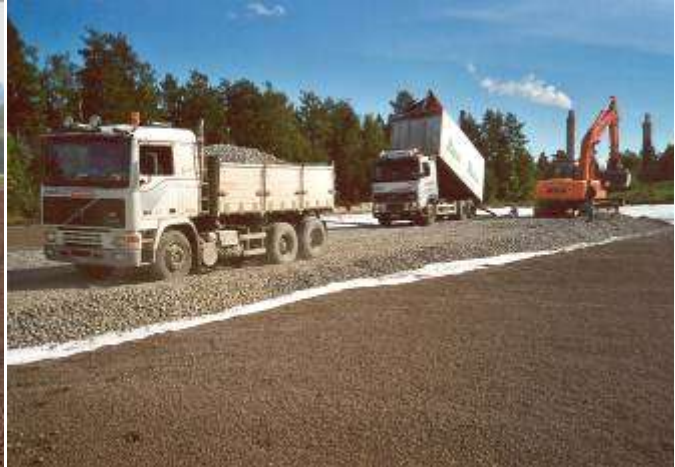
Figure 11 Access road on top of expanded clay LWA-fill
