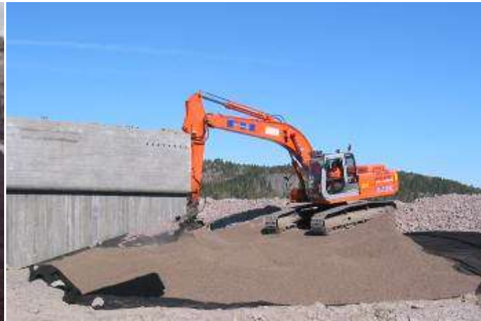
Figure 9 Spreading by a back excavator
