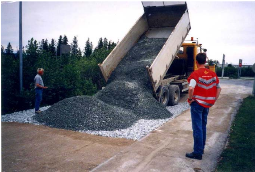
Figure 11 Construction of full scale field test
