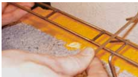
BI-binder legges rundt fugearmeringen
