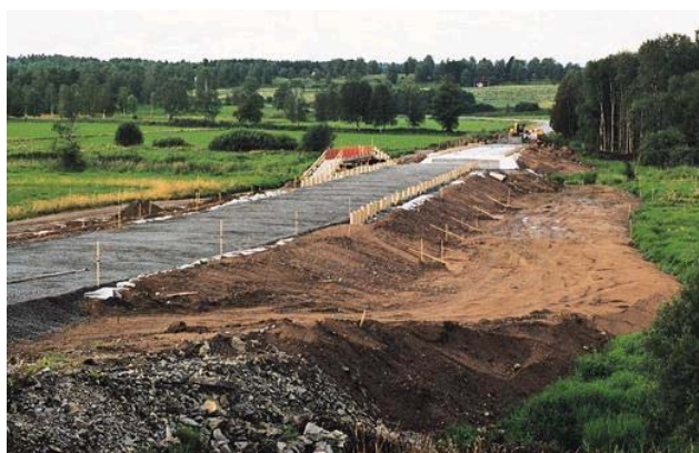
Figure 3.6 LLP-Light loadspreading plate
