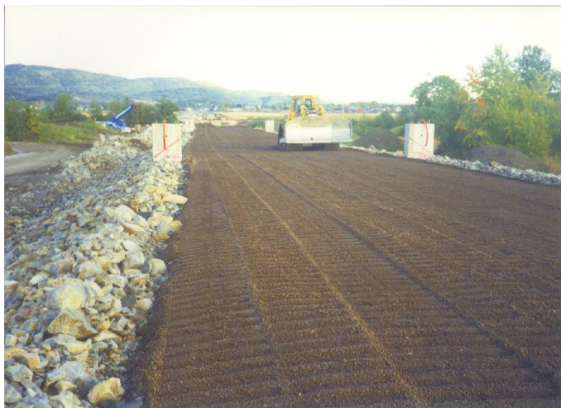
Figure 3.4 LWA as frost insulation in railroad embankment, Vestfoldbanen, Norway
