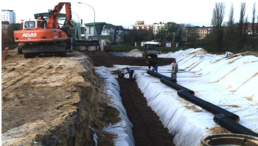
Figure 5.4 LWA in drainage ditch
