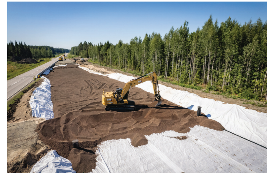
Leca LWA layer 1.3–3.3 m, enclosed in geotextile.
