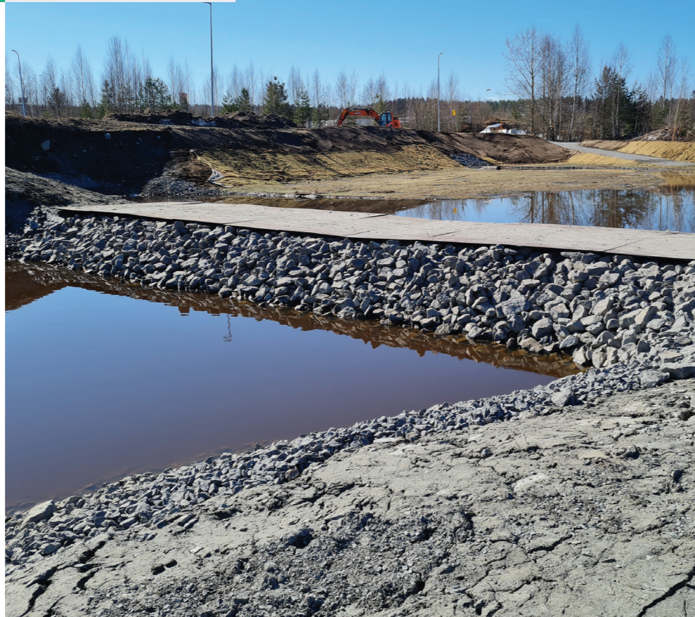
Completed dam filters water before discharge.
