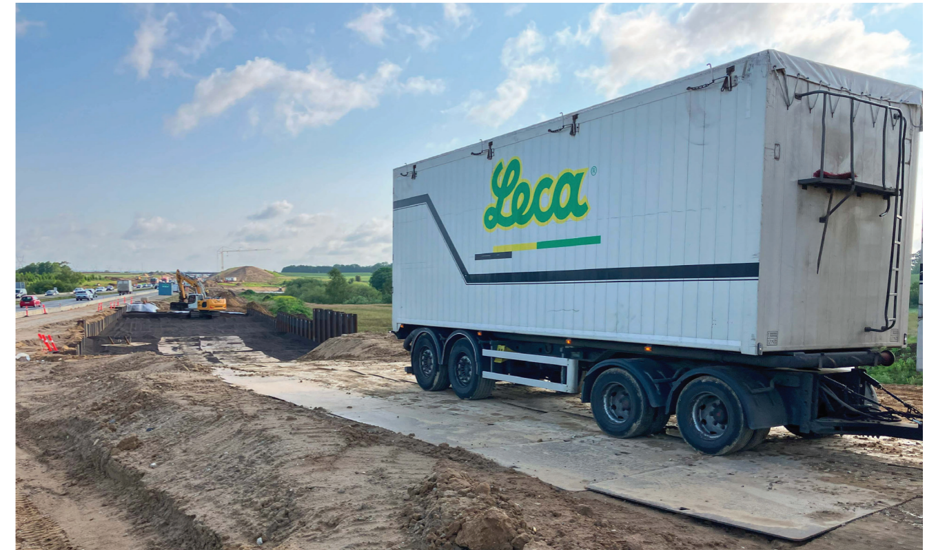
Delivery of Leca® lightweight aggregate for the E45 expansion. The material arrives ready for placement, ensuring an efficient construction process.
