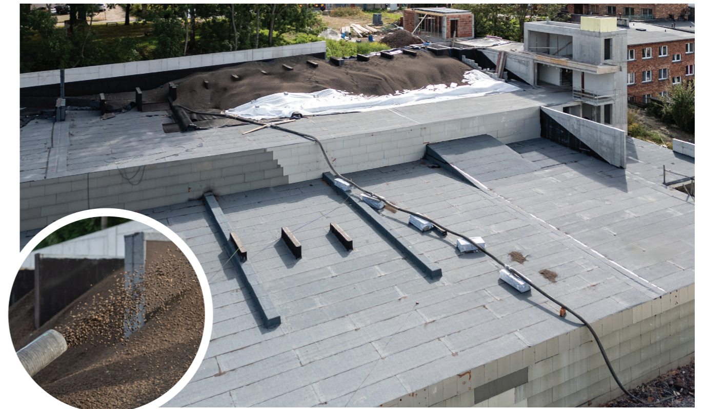
Leca LWA was pneumatically delivered directly onto the roof structure.
