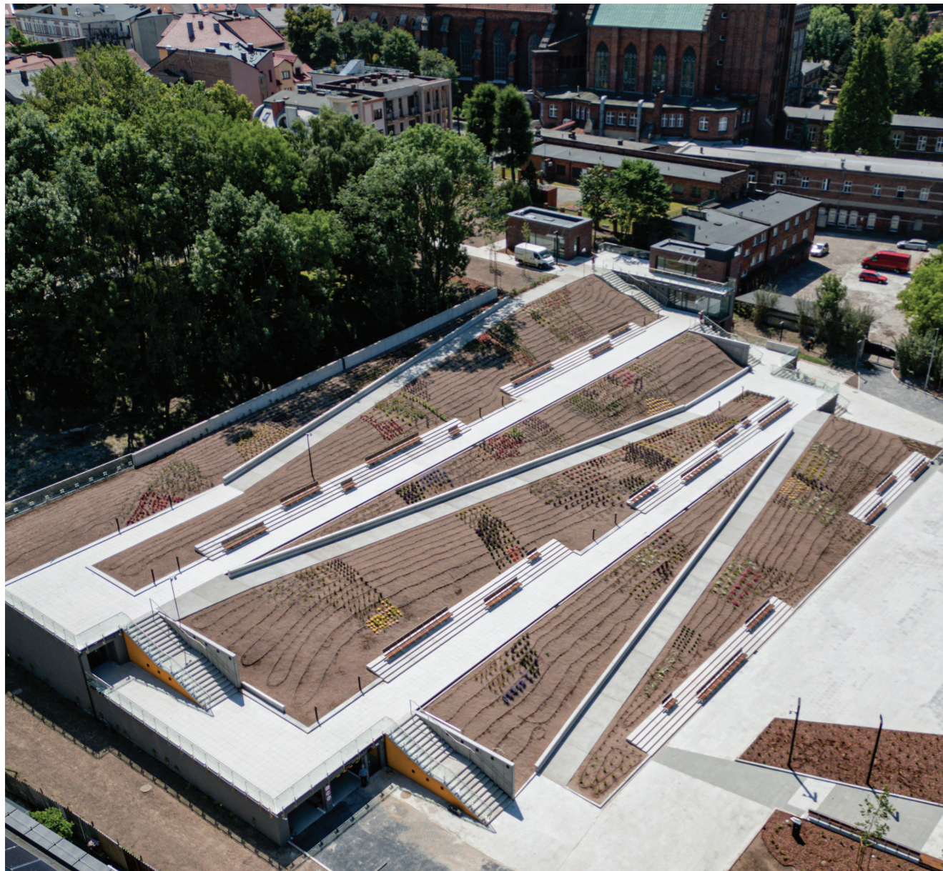
Leca LWA was selected for its reduced weight, minimal water absorption and excellent drainage capacity
