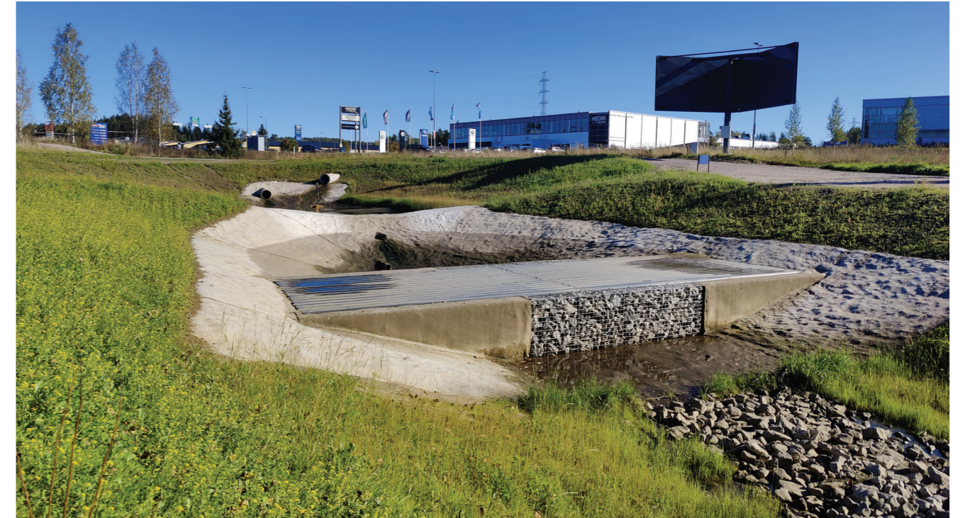
In Nikkilä, the filter dam completes treatment.
