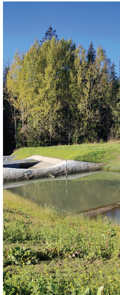
Filter dam integrated into a wider treatment chain.
