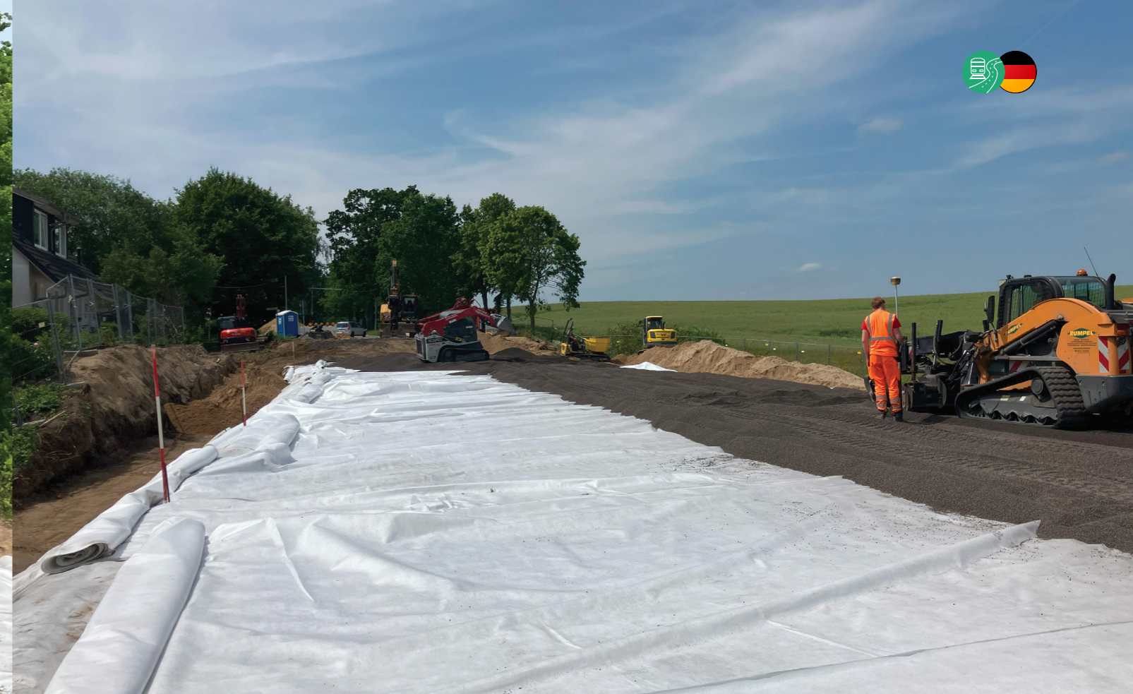
Leca LWA was enclosed in a geotextile
