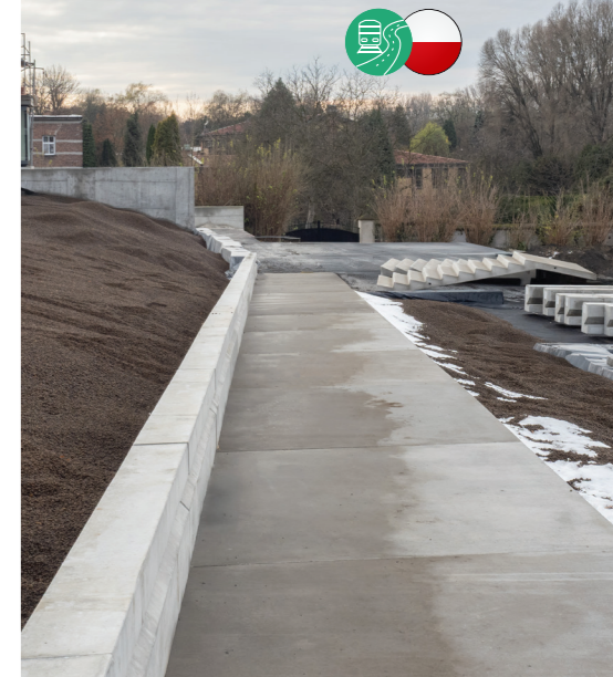
The new two-storey parking facility offers 142 parking spaces, electric vehicle charging stations, safe zones for cyclists, complete with bike racks and a service point.
