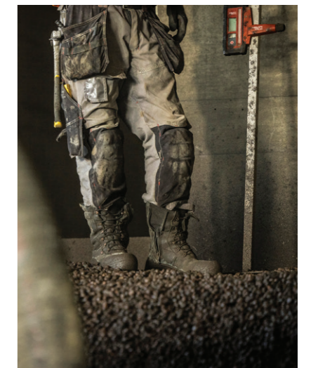
Leca blown into place, straight from the truck, fully compressed - no need for manual unloading, no problems to walk on and zero packaging.
