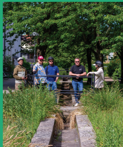
The channels in Augustenborg relieve pressure on old drainage systems by managing rainwater. Photo, Essi Malinen-Lallukka
