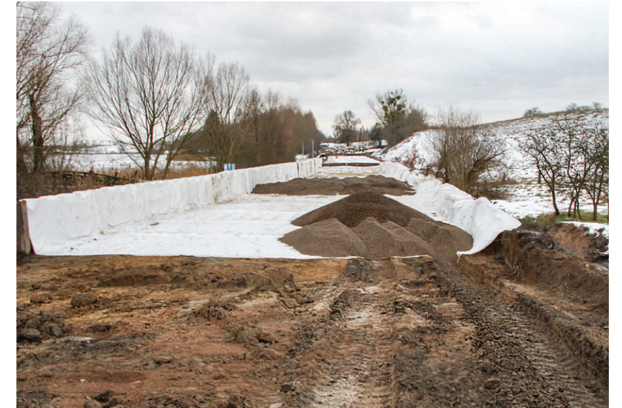
It was decided to use a geomattress made of Leca® GEOTECHNICAL EXPANDED CLAY 8/10-20RX."
