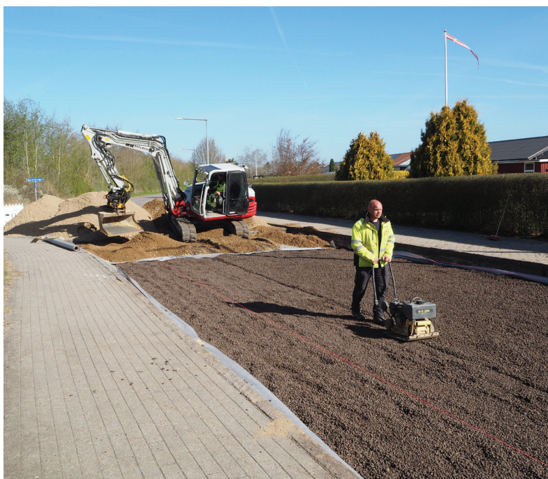
Leca LWA replaces sand as bottom protection
