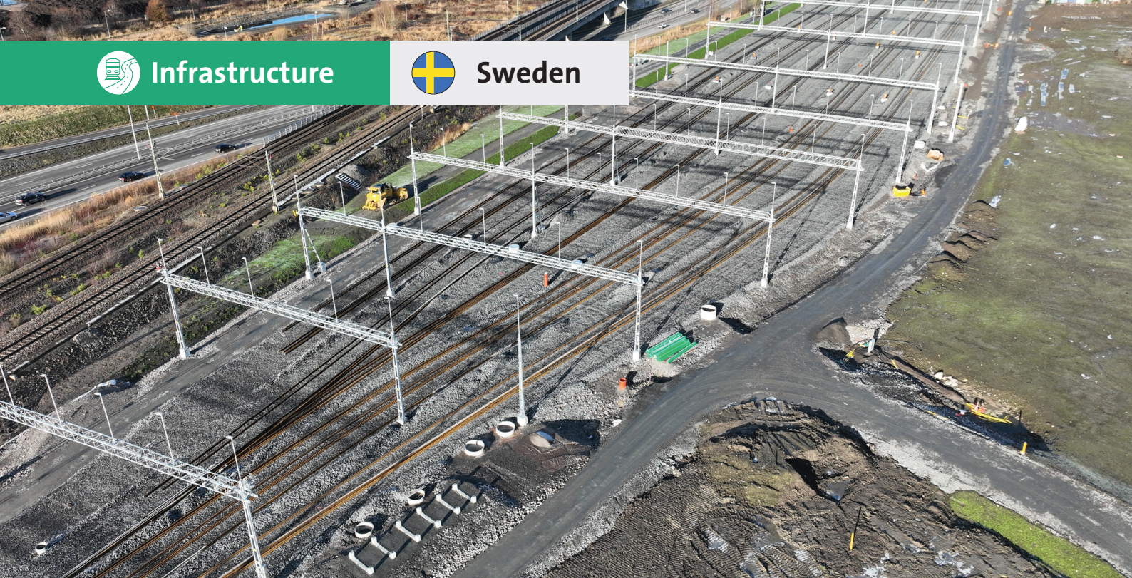
New stabling tracks taking shape – designed for increased capacity and future rail traffic. Photo Tim Cato, The Swedish Transport Administration
