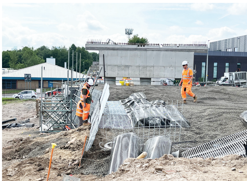
Lightweight fill required to reduce settlement risk and structural load on bridge abutments.
