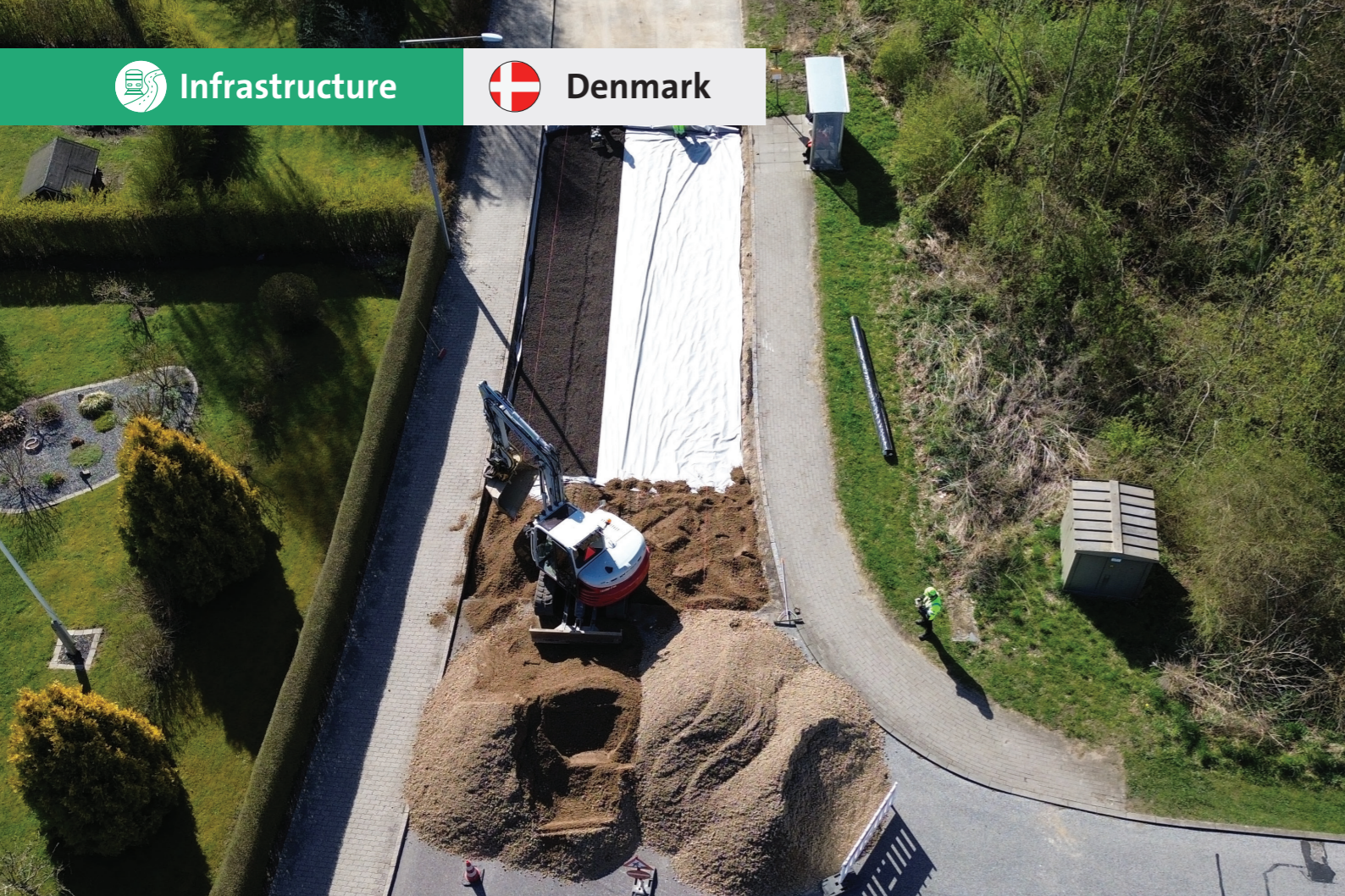
Fast installation and delivery make Leca LWA an obvious choice in infrastructure.
