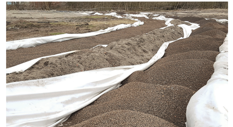
Compacted Leca LWA (8/10mm–20mm) in geosynthetic material forms load-reducing “expanded clay aggregate mattresses”.
