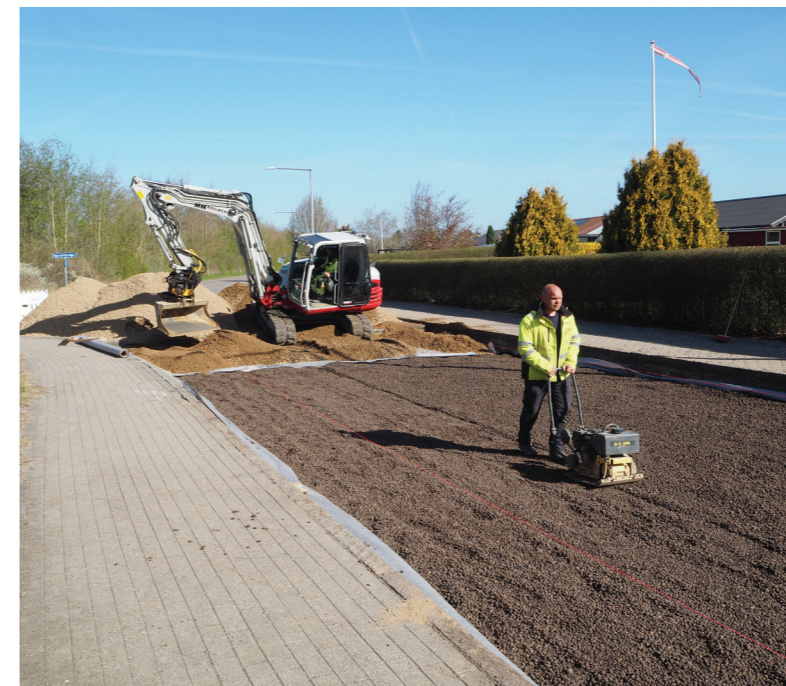
Leca LWA replaces sand as bottom protection
