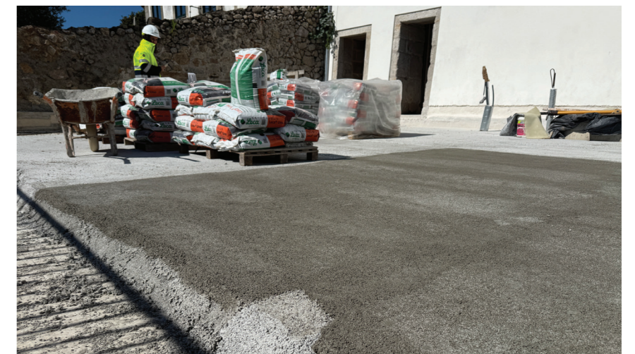
The terrace overlooking the River Douro — where Leca® Mix is visible in the image — will be the focal point of the hotel's leisure areas.
