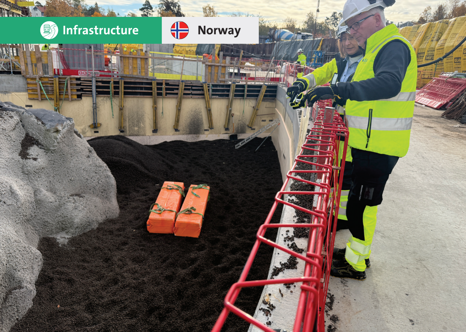
Representatives from Leca visiting the project site to inspect the installation of Leca® LWA, used to reduce earth pressure and improve safety and efficiency in a confined construction area.
