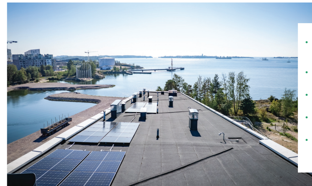
The completed roof integrates technical installations and solar panels within a lightweight and adaptable structure.
