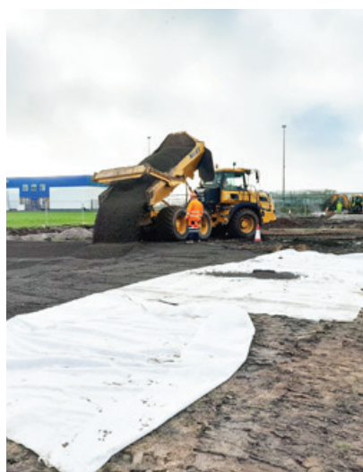
The presence of soft ground made conventional construction methods unsuitable for the project.
