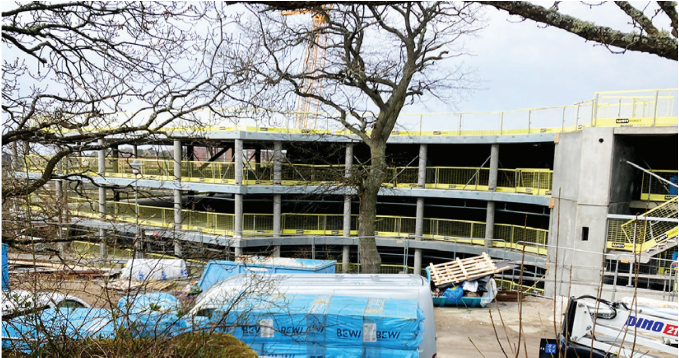
The parking structure was adapted to preserve the oak tree and protect local biodiversity.
