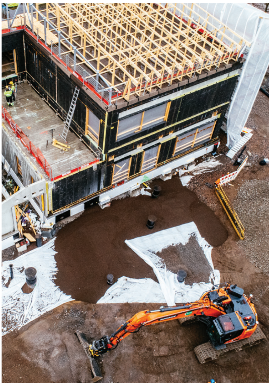
Over 2,000 m 3 of Leca LWA was used for the lightweight fills at Puotila School.
