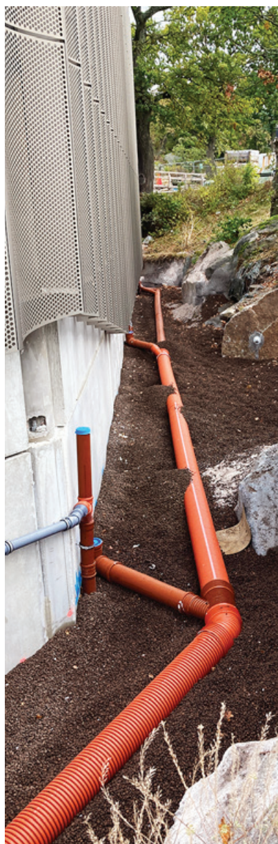
Leca LWA is used as backfill to stabilize the porous rock next to the building.
