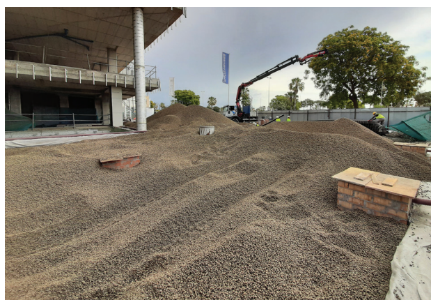
The lightweight fill, with thicknesses ranging from 0.8 to 1.5 m
