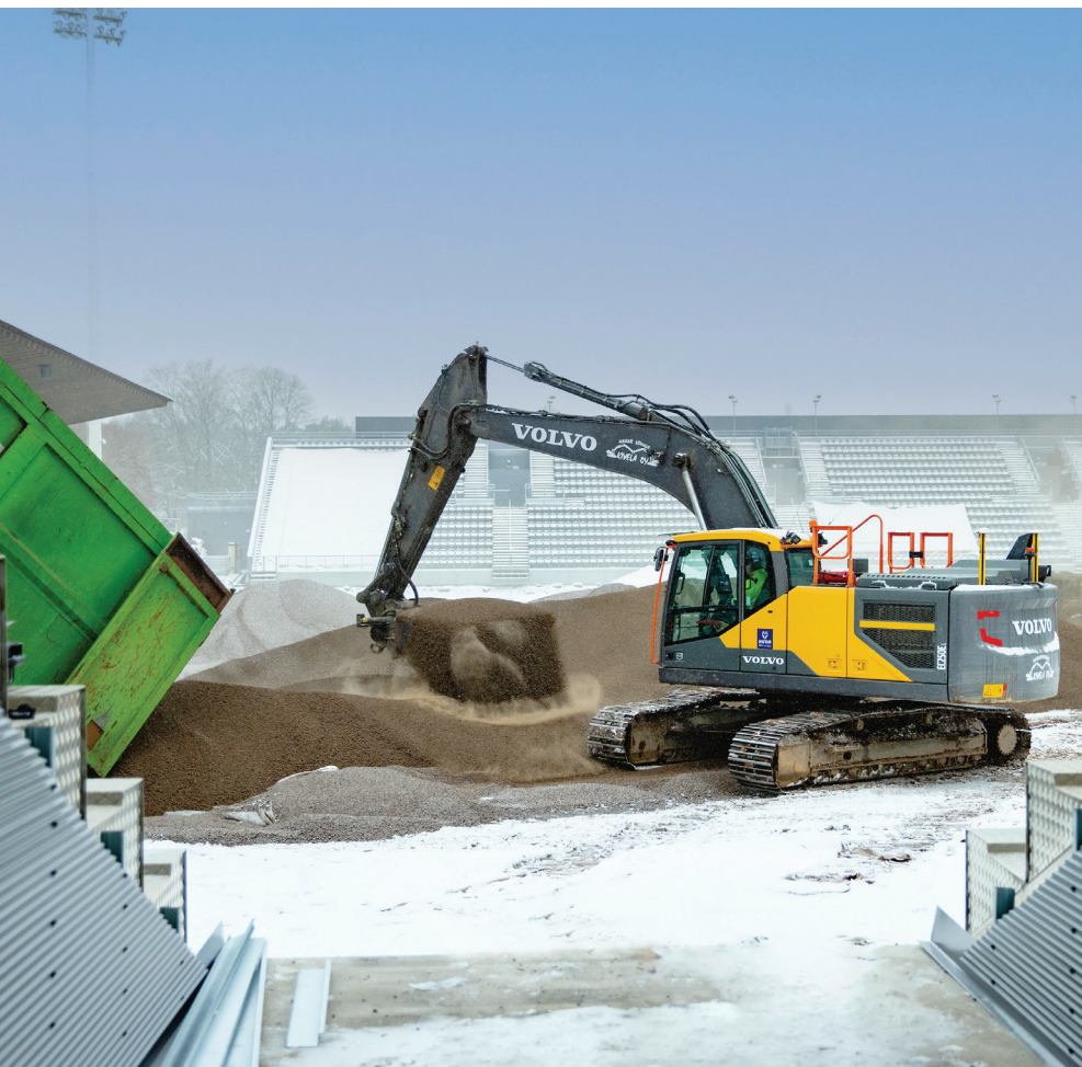
A 10-30 cm layer of Leca LWA was added on top of the old lightweight fill.
