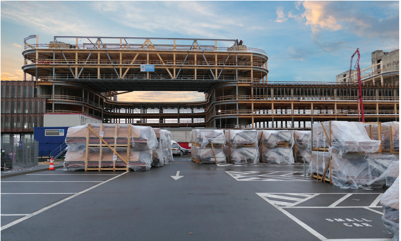
The Skypark Business Centre at Luxembourg's Aitport is currently the largest timber construction in Europe
