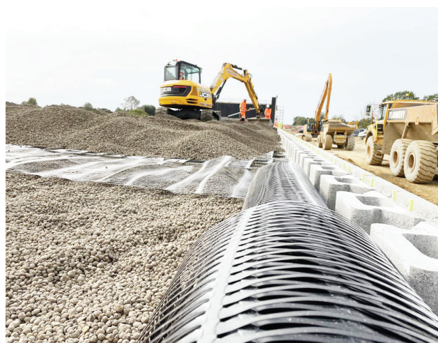
Innovation Meets Infrastructure: The Synergy of LECA LWA and the Tensar Grid System in Spalding
