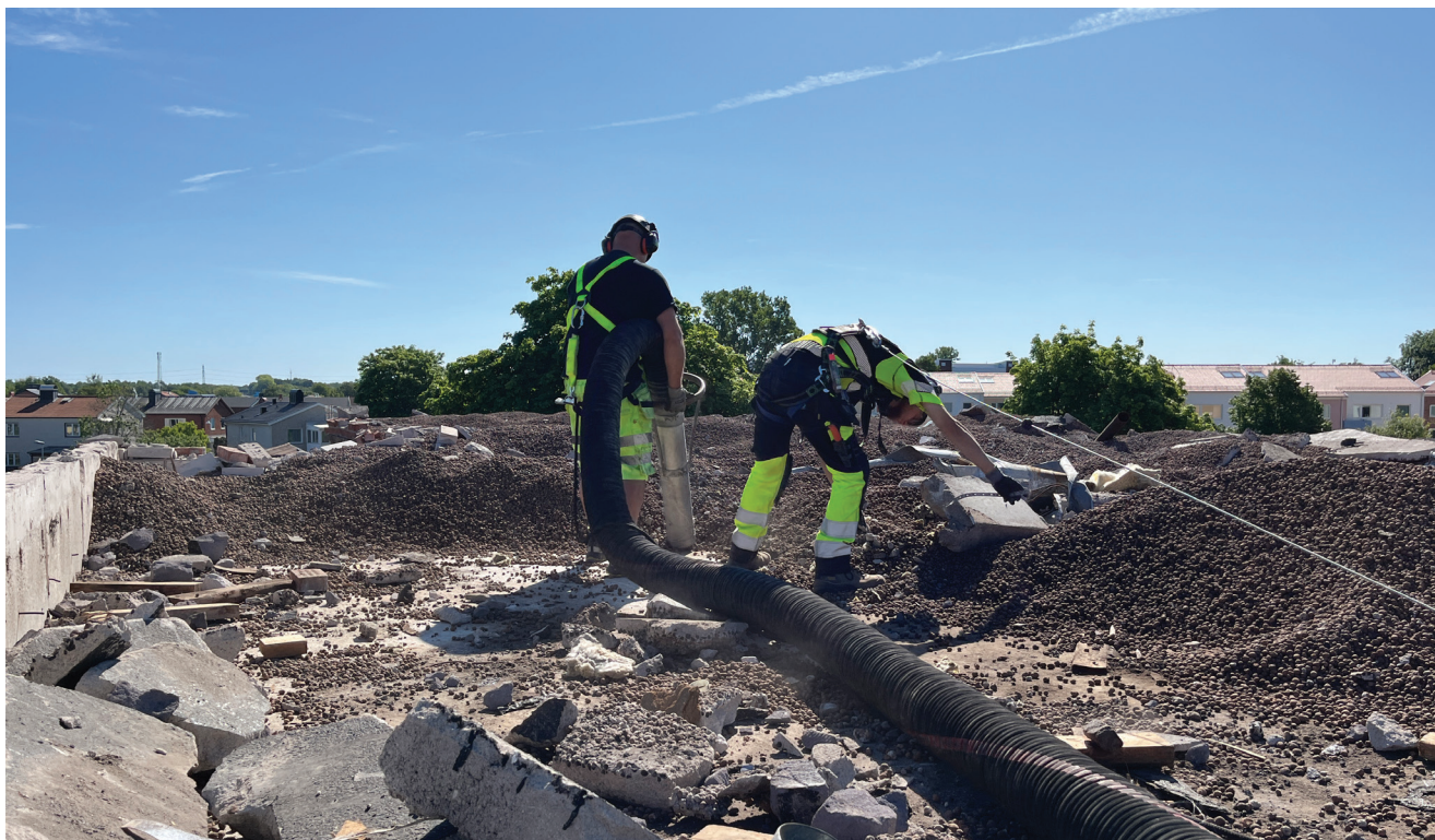
The lightweight aggregate in the roof from the 60's was analyzed and could be reused.
