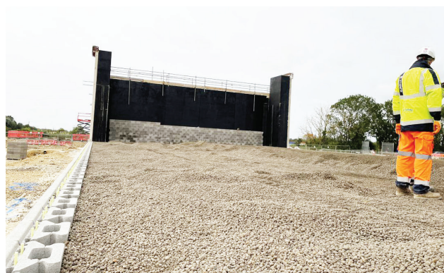
The use of LECA LWA in areas with poor ground conditions near waterways has proven to improve ground stability
