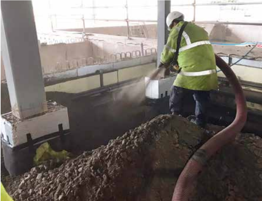
Leca LWA had the structural properties sufficient to take loading of a 150mm thick concrete floor slab
