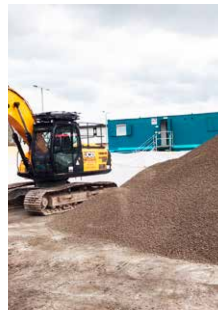
Leca LWA saved potentially 10+ days on programme plans and had the increased benefit of enhancing the thermal values of the pool tank
