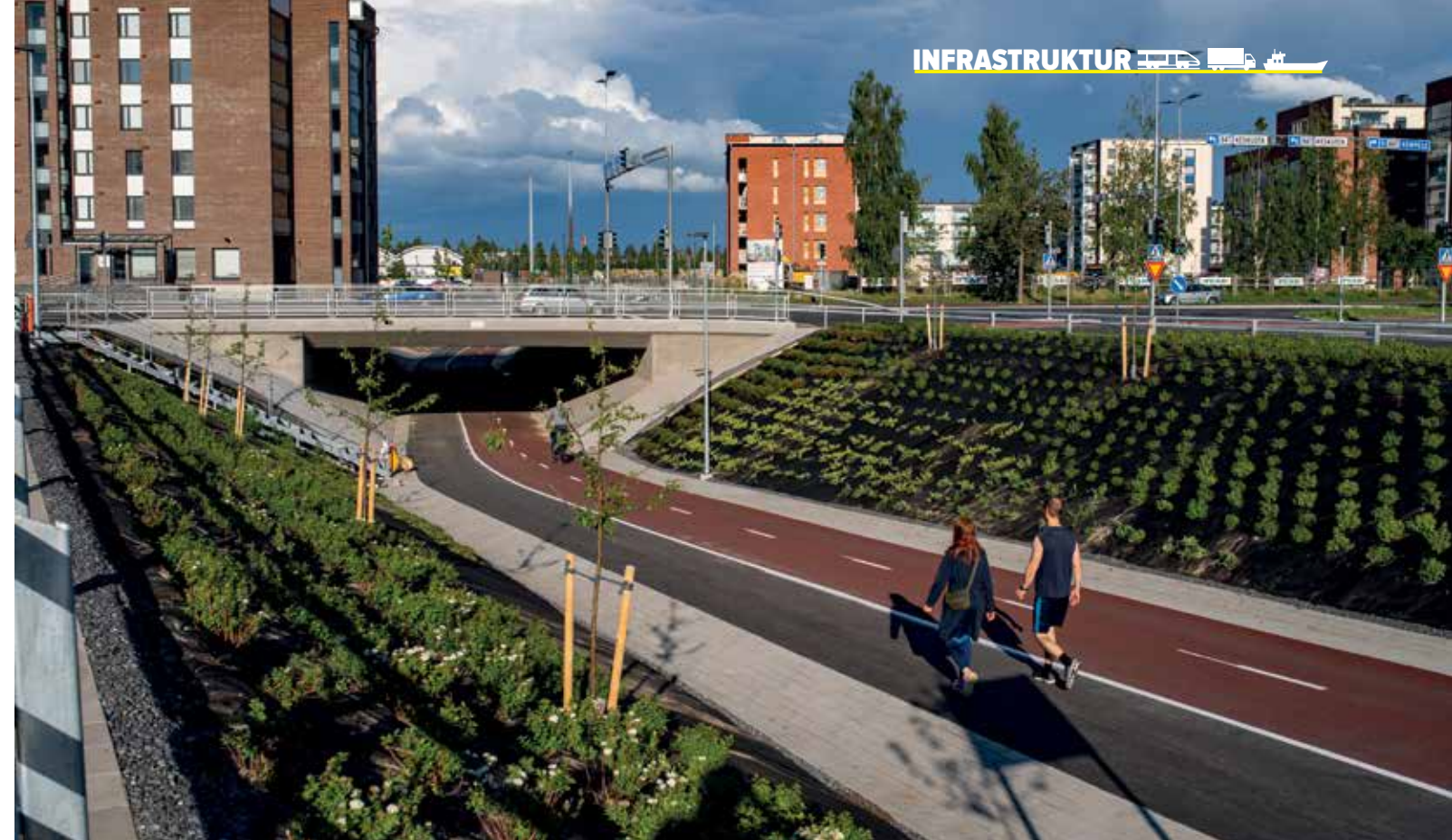
Rautionpolku-undergangen sto ferdig i november 2019.
